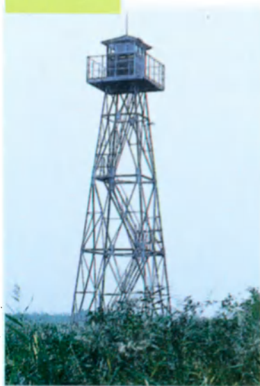
This watchtower, a vestige of the iron curtain, is now used for bird-watching.
