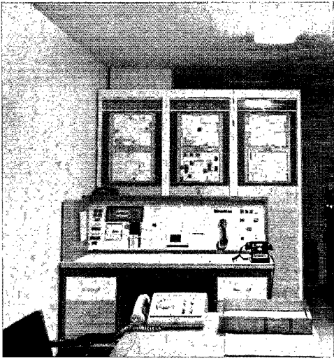
28. FINE ARTS GALLERY, Montreal. View of security and fire and smoke detection controls, with related equipment in guard-room.
