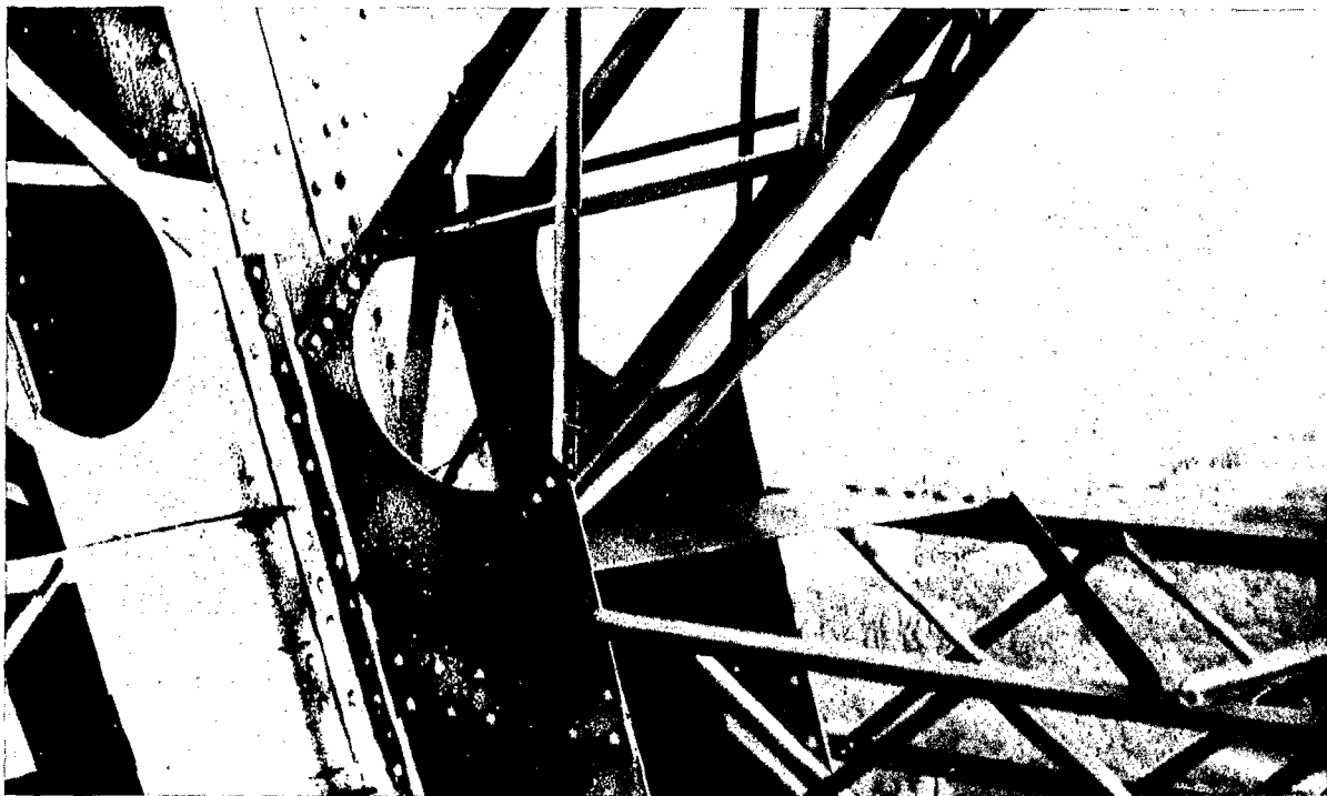
France. 'La Tour Eiffel': Photographic work by a 15-year-old student.
