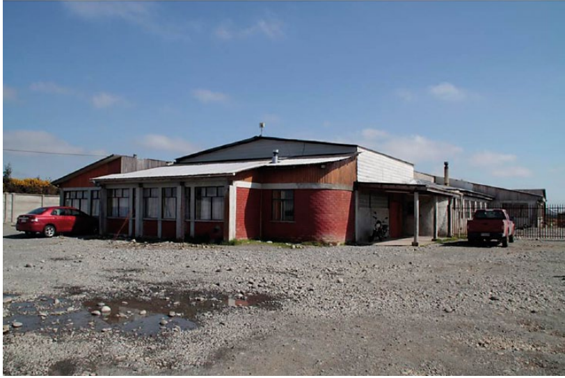
3 Urban school, 196 students: Los Alceres, 3000 inhabitants, near Puerto Montt city, approximately 600 miles south from Santiago. © Photograph: Josefina Buschmann.
